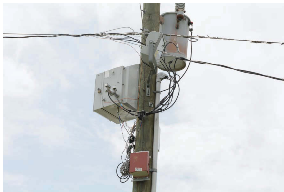
FIGURE 8.23 Secondary voltage regulator installed on a feeder (mounted below distribution transformer). (© 2016 Gridco Systems. All rights reserved.)
