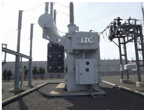
FIGURE 8.3 Photograph of a distribution substation power transformer with an LTC.
